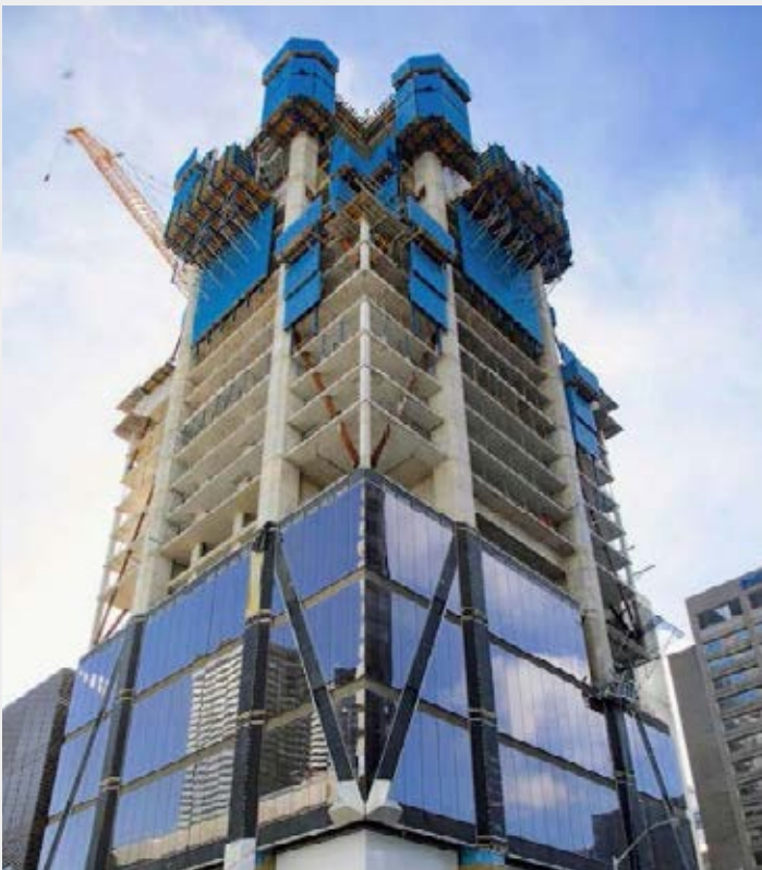
Fig. 17: Exterior view of the tower early in construction showing the ACS at the top, hanger columns and envelope progress above the ground floor retail. The RCS system was not yet installed in this photo
